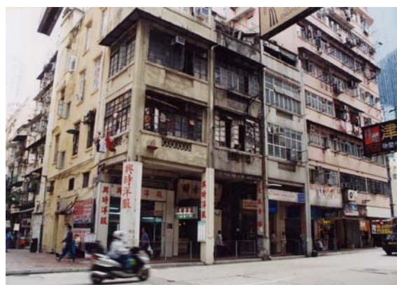
Figure 3.2 Three pre-war tenement houses at 186 - 190 Queen's Road East, Wanchai
