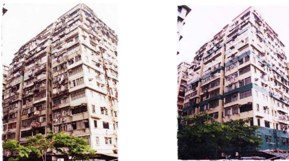
Figure 7.1 Chung Sing Building before (Left) and after (right)
