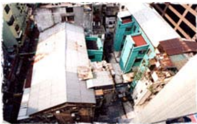
Bird's eye view of the site
