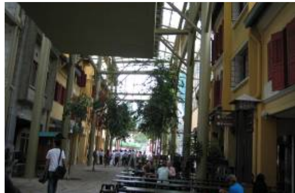
Figure 3.6 The open space within Far East Square covered by a glass and steel canopy
