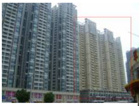
Figure 8.3. On-site relocation blocks (circled in red) for residents of Xian Cun (洗村), a town-village 244 .
