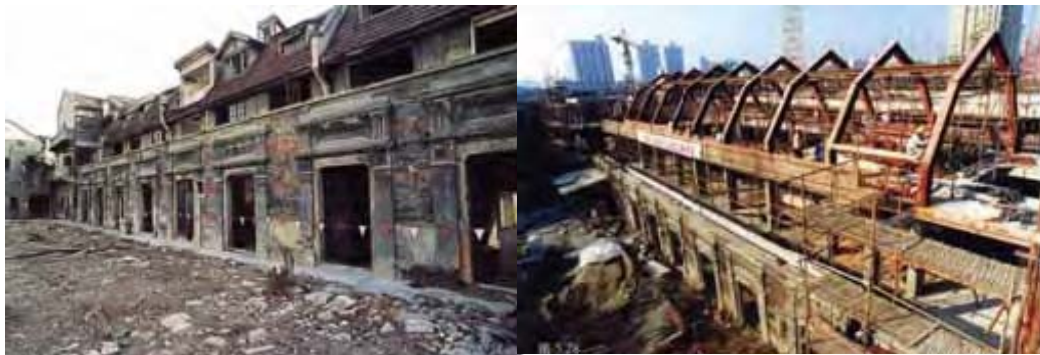
Figure 7.4. The original appearance of stone gate row and the new roof frames added in the renovation work of Shikumen houses.
