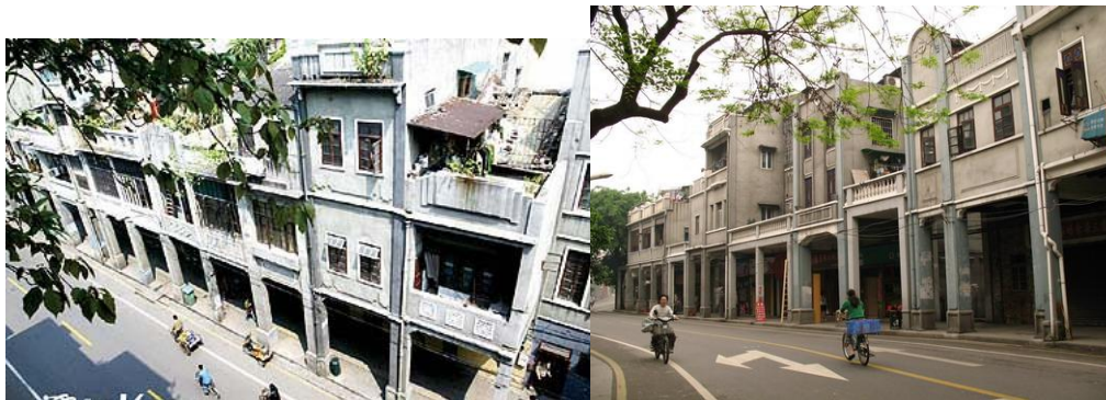
Figure 8.5. Cantonese style shop-house in Enning Lu, Li Wan District 253
