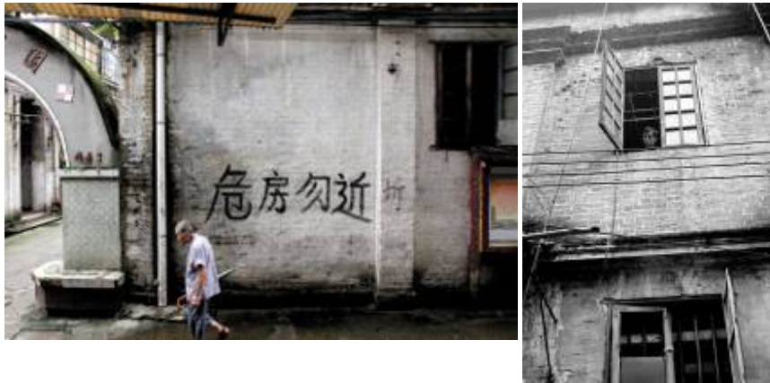
Figure 8.1. Dangerous and dilapidated buildings
