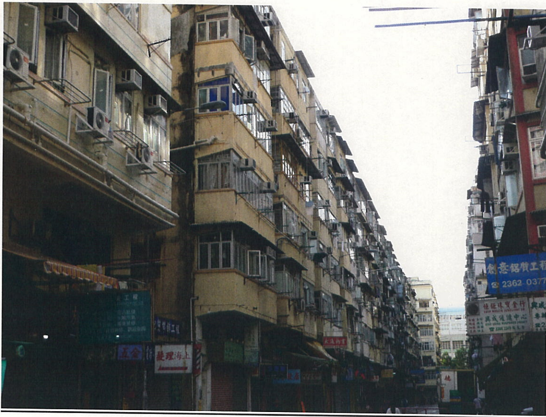
Old Buildings in Ngan Hon Street (Prop. Redevelopment Site B)
